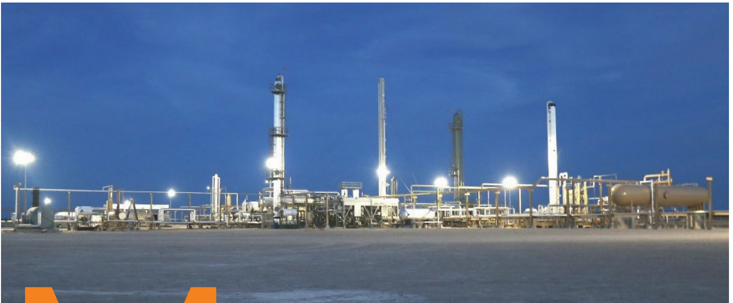
Processing Plant in the Delaware Basin
