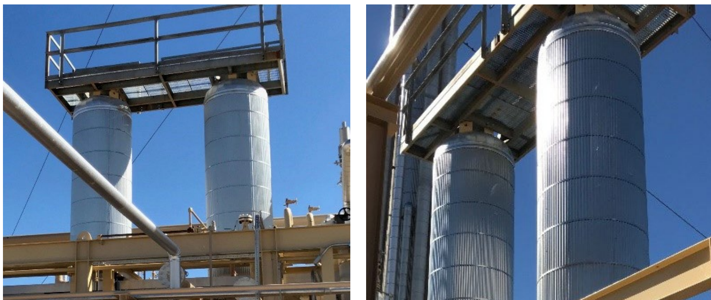
Figure 1: Mol Sieve System in a Cryogenic Plant
