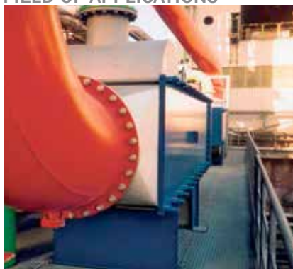
Low pressure vapour condenser
